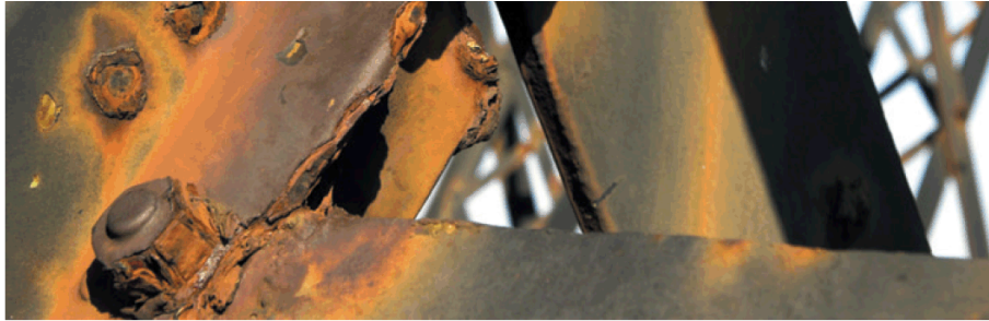
Corrosion costs around US$4 trillion a year globally.
